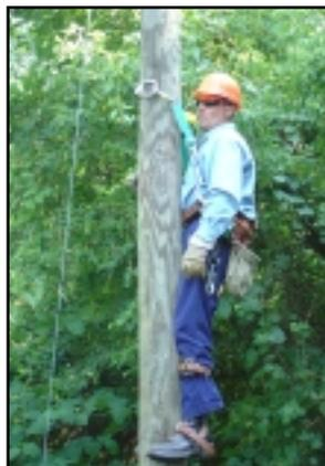
the belt's cinching action around the pole. When adjusted properly the BuckSqueeze limits the user to a fall of just a few inches. It is an enhanced work positioning device that, if used properly, will prevent a fall off the pole.
