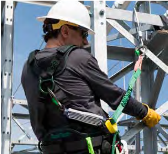
Climbing angle iron using the Versa-Yard™ and a BuckTech™ harness.
