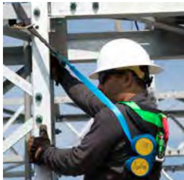
Using Dual Tie Back BuckLimiter™ with the BuckArticulator™ harness.
