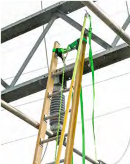
Installing stabilizer strap of BLT over trussing to access the buss.
