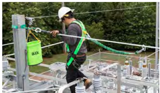
Shown below, the Buckingham Horizontal Lifeline System provides fall protection for users working on gang operated three-phase air switches.
