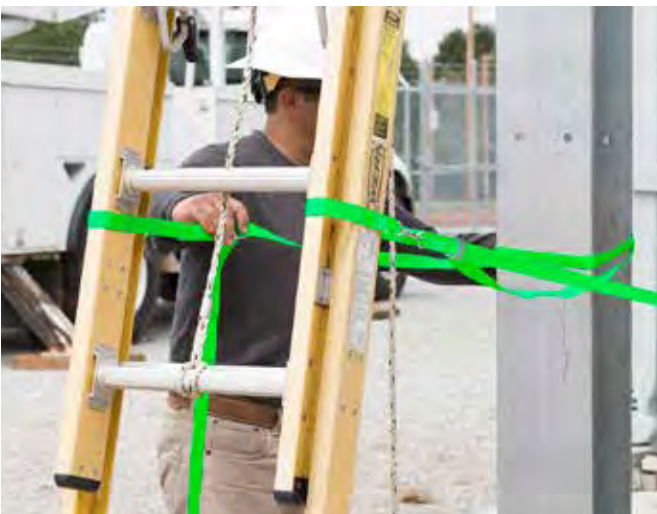
Installing stabilizer strap of Ladder Lock (model 355B) to steel.
