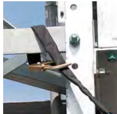
Close up of tie-back snap with wear guard.
