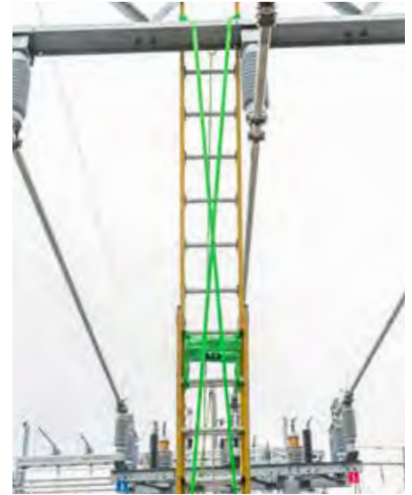
Rear view of BLT attached to trussing.
