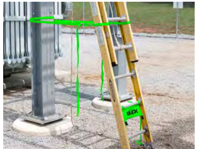
Ladder Lock (model 355B) used to secure ladder to steel prior to working.
