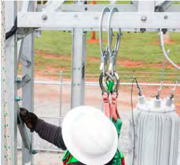
Big BuckSnaps™ attached to the Versa-Yard™ and attached over angle iron.
