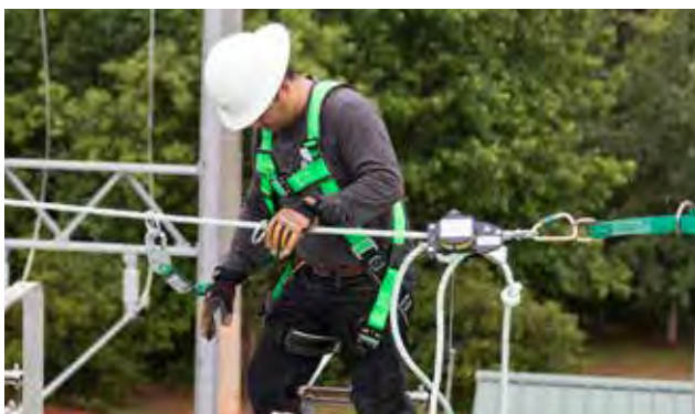
Shown below, the Buckingham Horizontal Lifeline System provides fall protection for users working on gang operated three-phase air switches.
