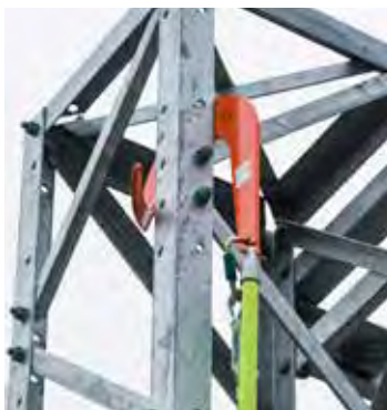
2. Secure the BuckHook™ onto structure.
