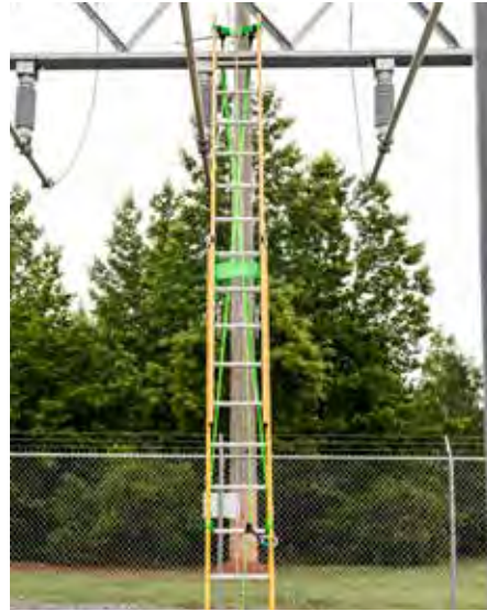
Front view of BLT attached to trussing.
