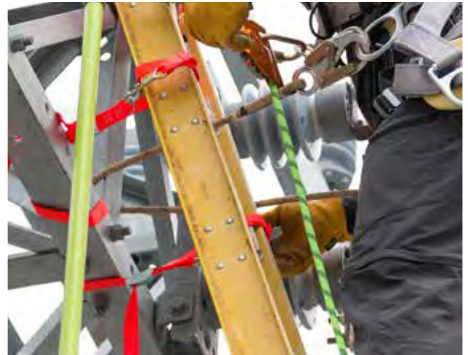
Ladder Lock (model 355T) used to secure top of ladder prior to working.
