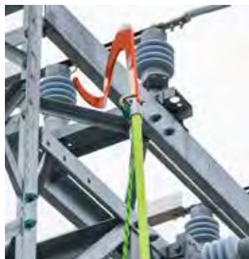
1. Lift the BuckHook™ w/lifeline to desired point on the structure.
